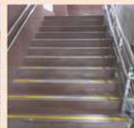
Staircase (Colour strips, handrail)
