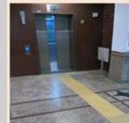
Lifts (Braille, Audio, Warning tile)
