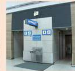
Drinking Water Facility
