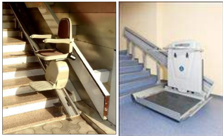
Figure 7-18: Platform chair lift and platform lift
