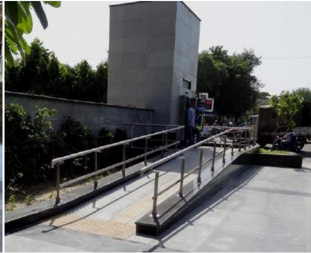
Figure 11-5: Lift access to subway crossing
